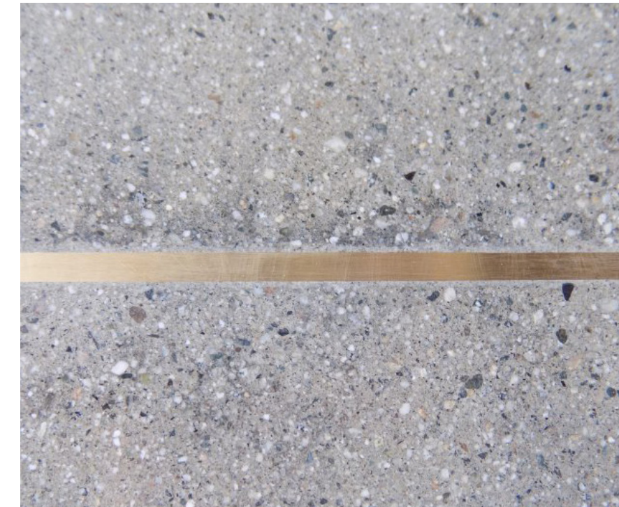
Site Paving with Brass Inlay
