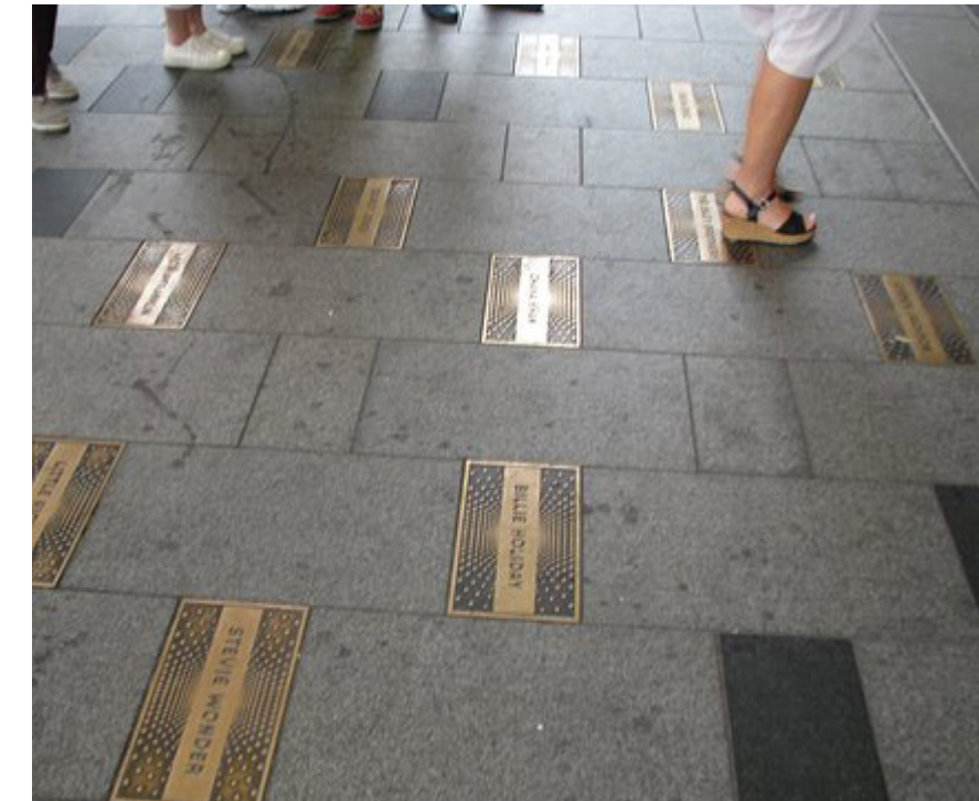
Site Paving with Brass Inlay
