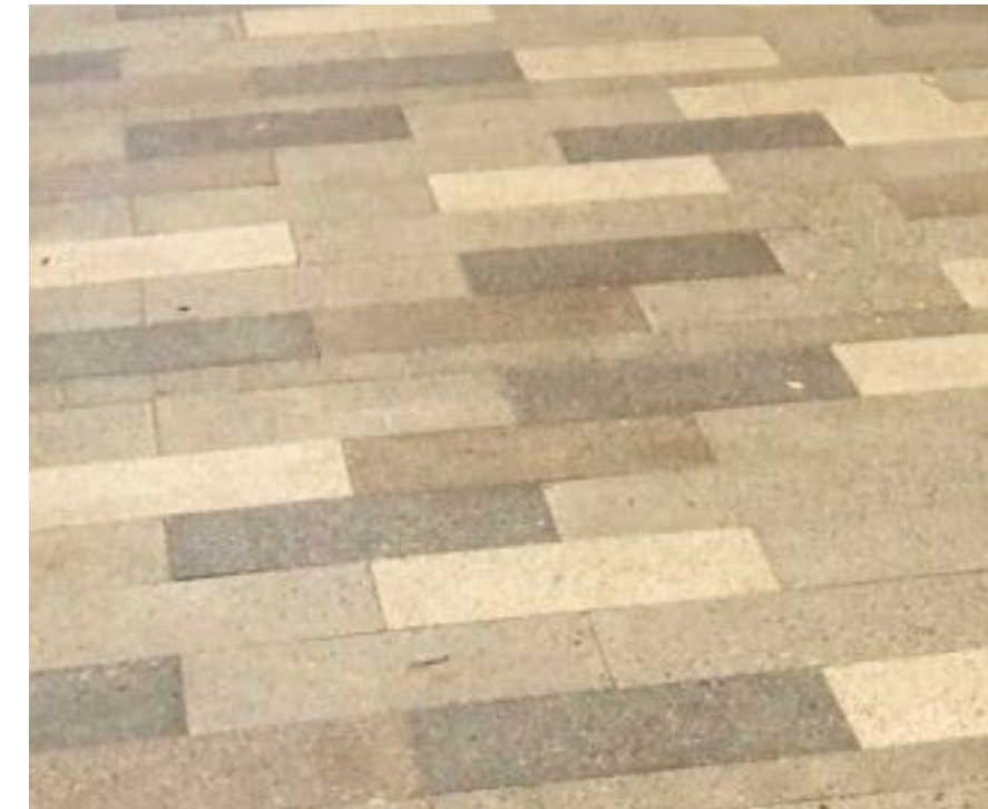
Street Paving 2 (Burlingame Ave Paver)
