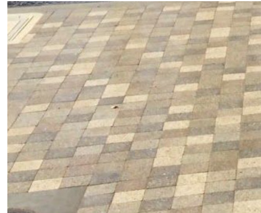
Street Paving 1 (Burlingame Ave Paver)
